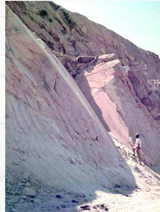
A wedge failure controlled by intersecting structural features in the rock mass
